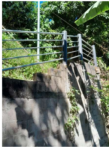
installation of lamp near new staircase.
