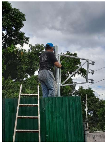
Installation of pole to support electric power cables near church.
