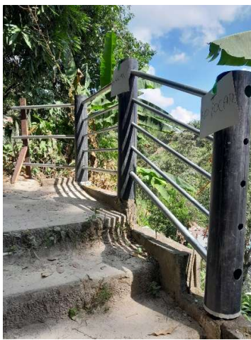
Railings erected by residents beside concrete staircase.
