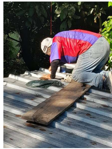
mending the Community House roof.
