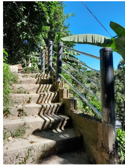
concrete staircase provided by City Hall.
